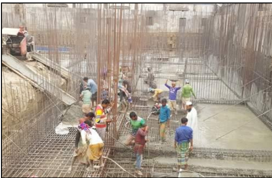
Fig 1: Raft foundation
