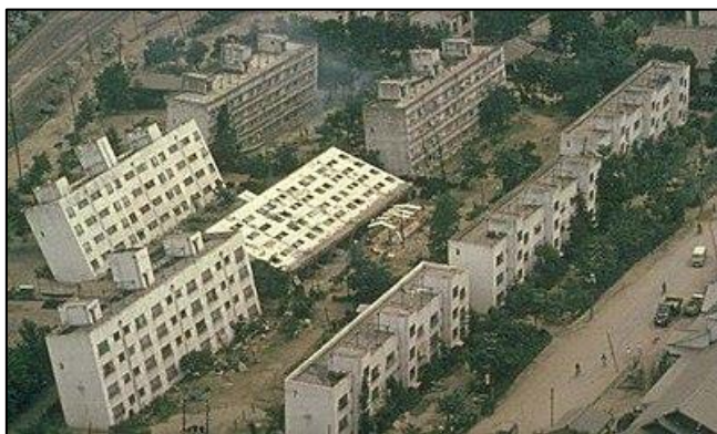
Fig 1: Some effects of liquefaction
