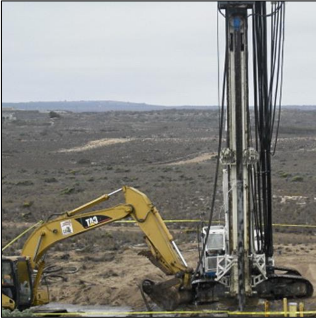
Fig 5: In-Situ Stabilization
